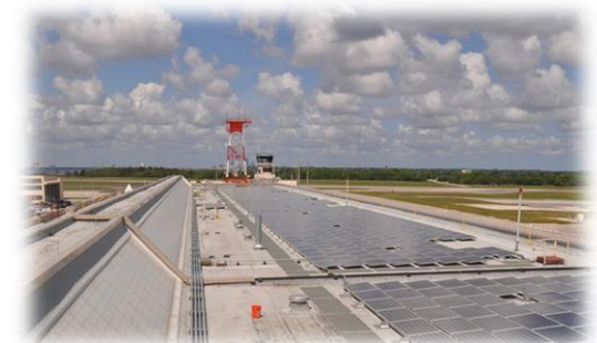
Solar on Hangar Roof
